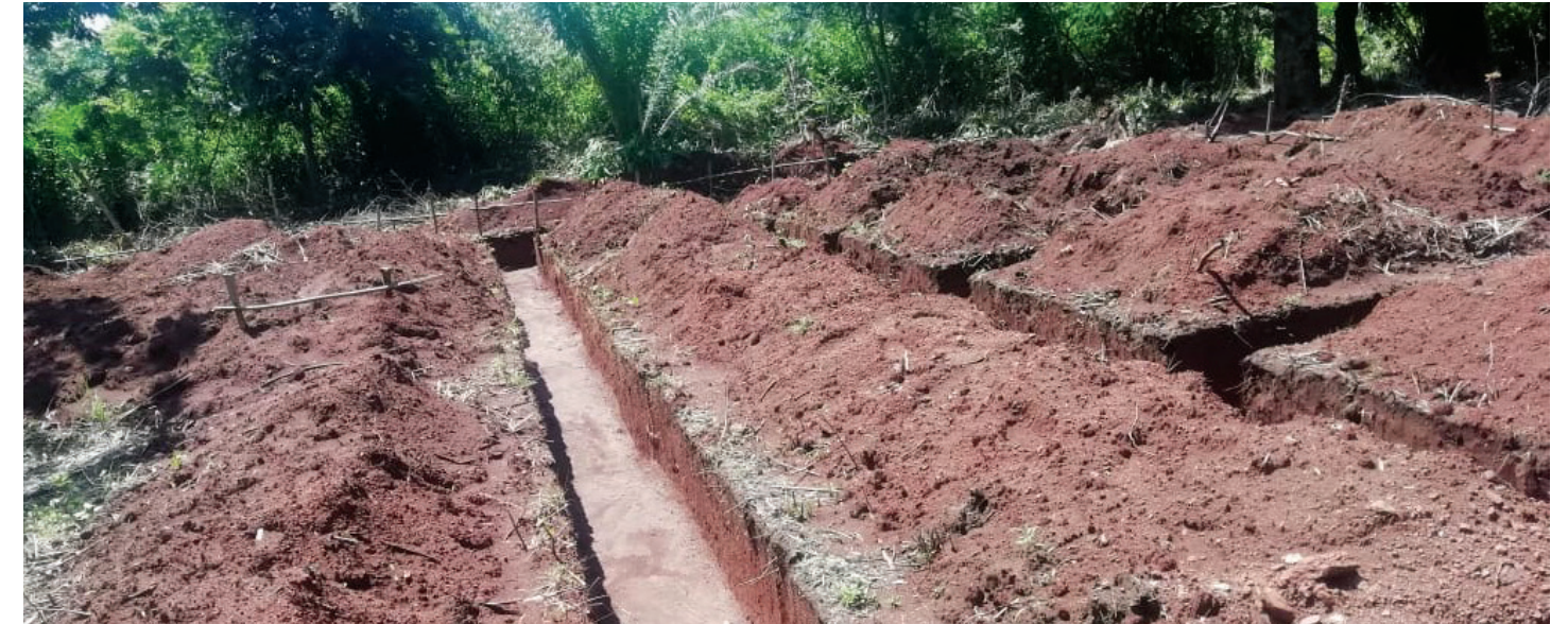
Breaking ground. Laying foundations for the new health clinic.
